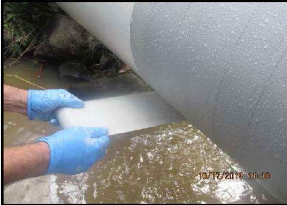
9. Immediately upon completing the installation (or at a hold point), wrap 4-6 layers of constrictor wrap.
