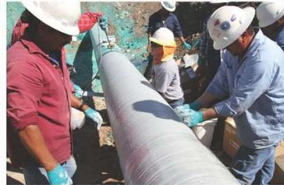
**A+ Wrap** is a high strength fiberglass composite pre-impregnated with moisture cured polyurethane resin. It is designed for simplification of installation for restoring the structural strength of degraded pipe with varying geometries. It is also able to be used for pressure containment under certain circumstances.
