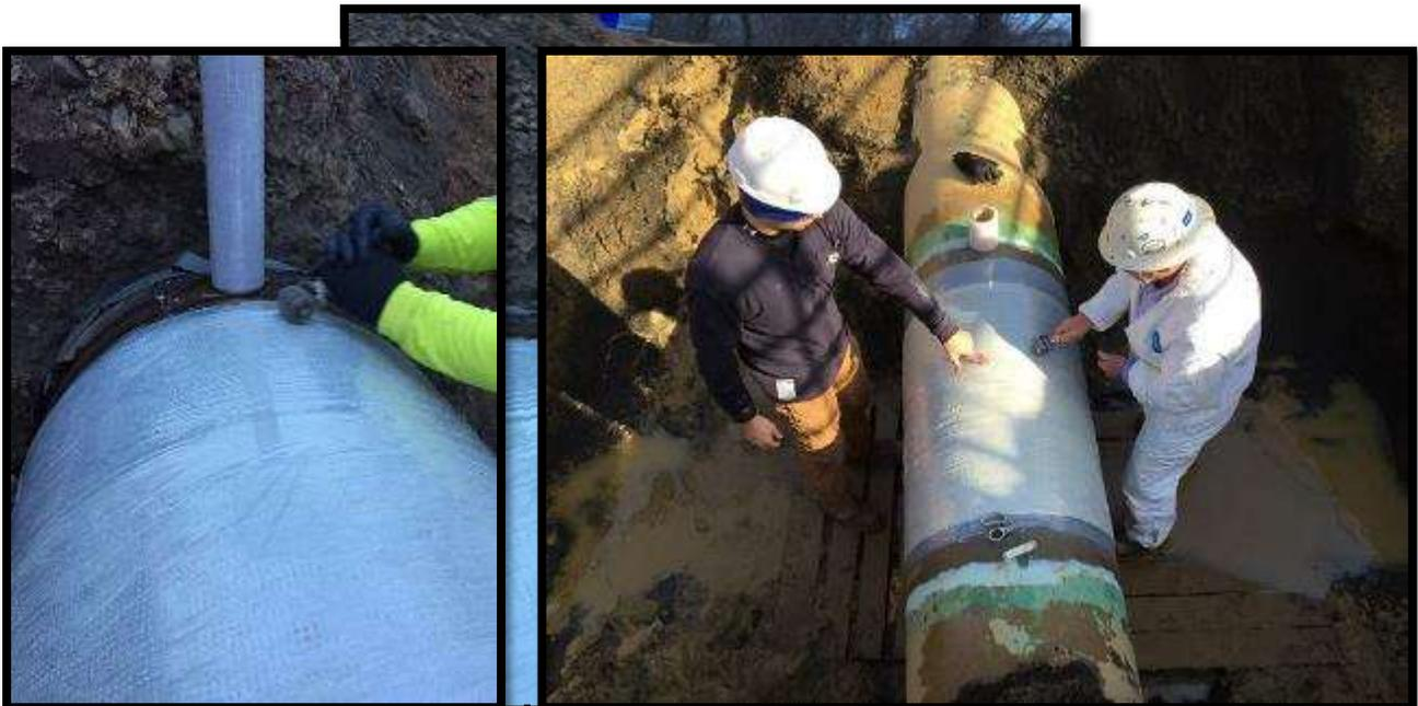
10. Immediately perforate the constrictor wrap to allow for out-gassing and de-bulking.
