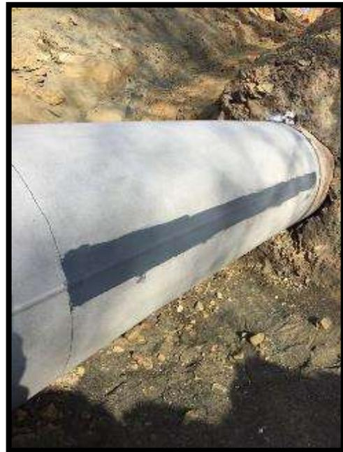
4. Mix and apply specified Load Transfer Filler materials over all defect and tented areas (i.e. welds), trying to return the pipe to a near-net profile. Smooth to pipe as needed.
