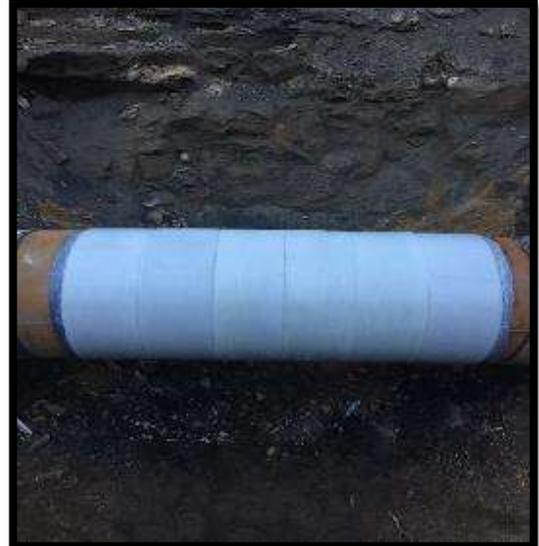
12. Top coat the repair if required (a top coat is always recommended over our repair systems).
