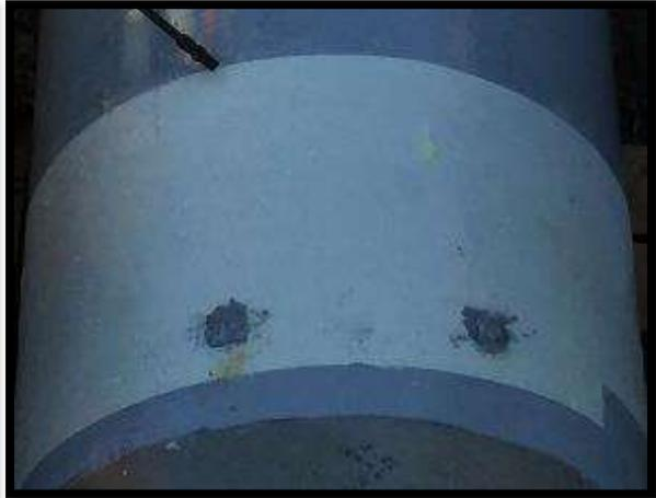
8. Continue wrapping per installation method. Once two layers have been achieved, ensure that constant, uniform tension is applied to the roll.
